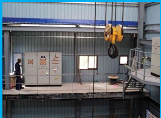
Installation of Control Panels
