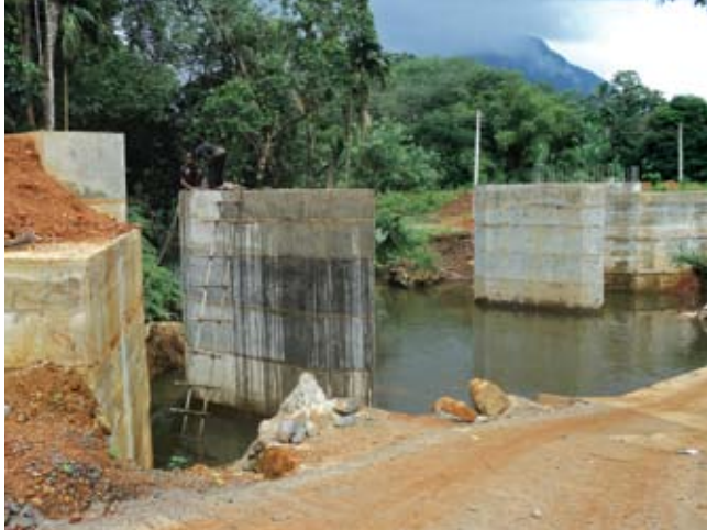
Construction of Bridge at Madugeta Village
