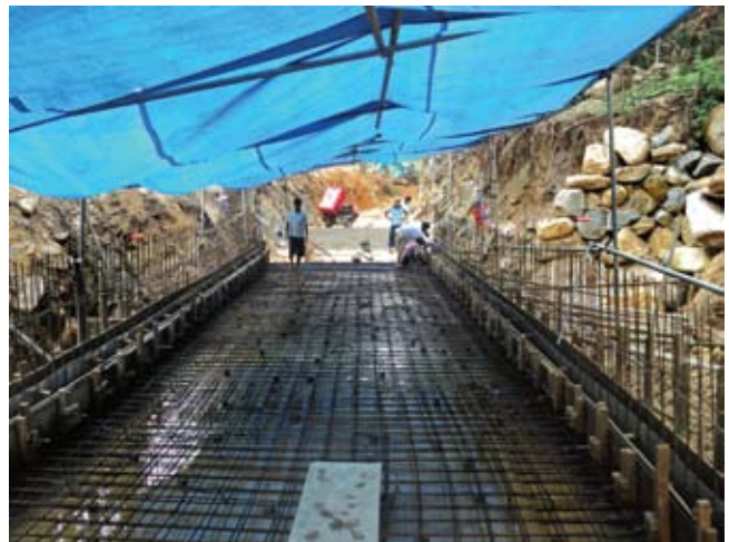
Fixing of Reinforcement at Channel Section
