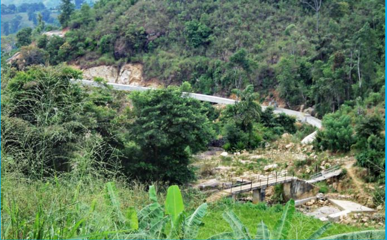
Completed Channel Section
