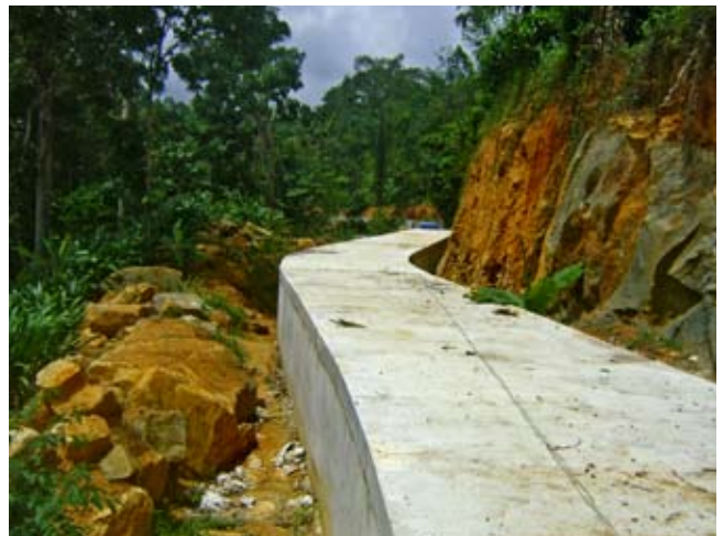
Completed Channel Section
