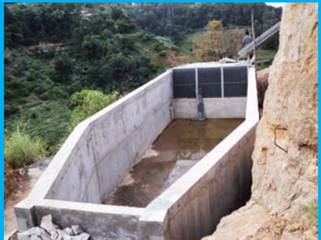
Completed Forebay Tank
