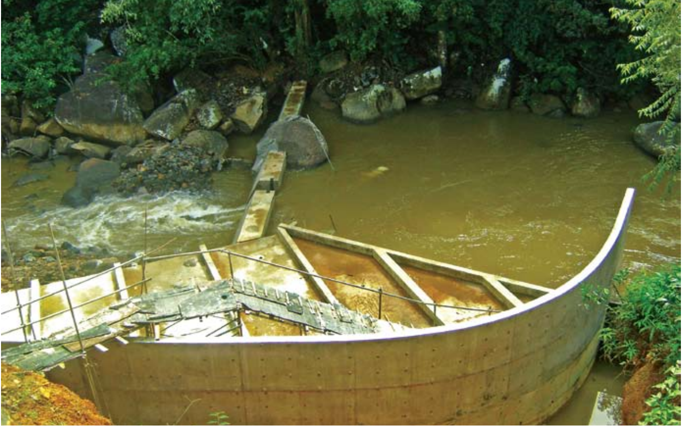
Completed Weir and Intake
