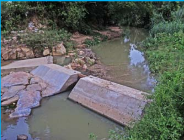
Completed Weir Section
