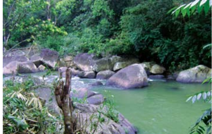
Weir Location at Wembiyagoda MHPP
