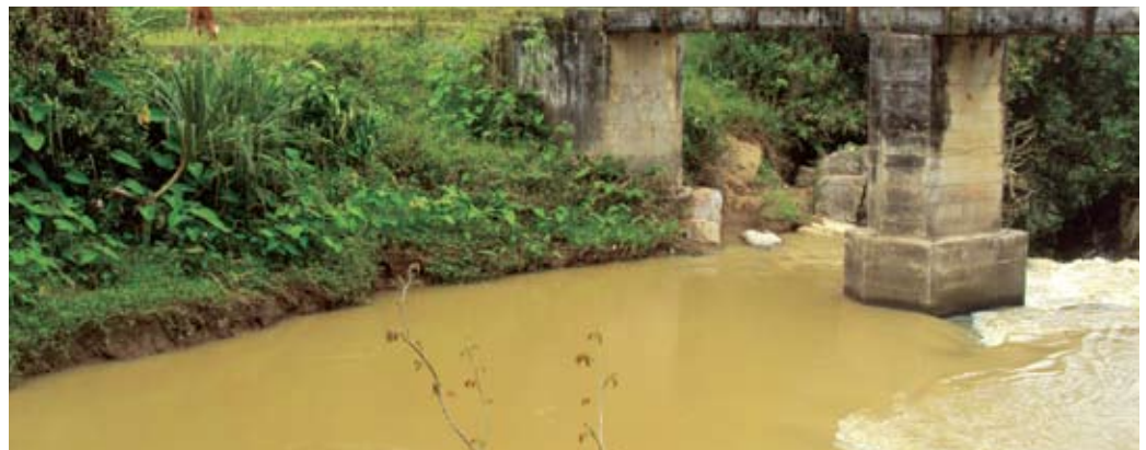
Weir Location at Hal Oya MHPP
