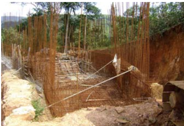
Construction of Forbay Tank at Ethamala Ella Mini Hydro Power Plant
