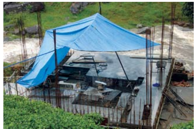
Power House Work - Sheen Mini Hydro Power Project
