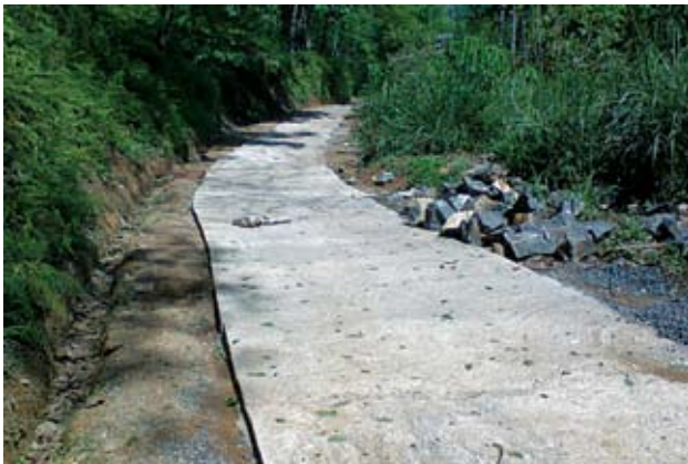
Construction of Access Road - Banagoda
