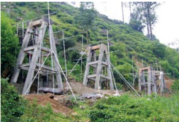
Construction of Penstock Supports - Sheen Mini Hydro Power Project
