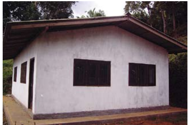
Construction of Sudagala Rahula Maha Vidyalaya Library - Banagoda
