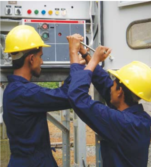
Maintenance of HT Breakers - Batatota Plant
