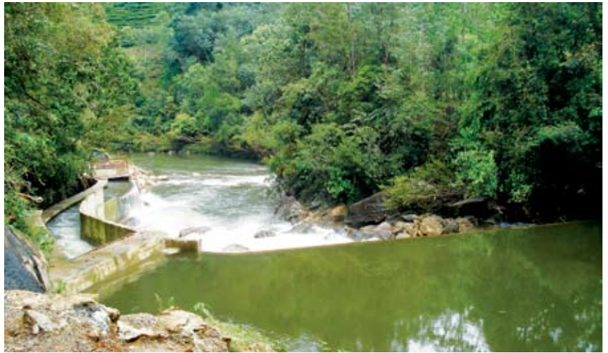
Intake and weir 'Flow diversion' - Batatota Plant
