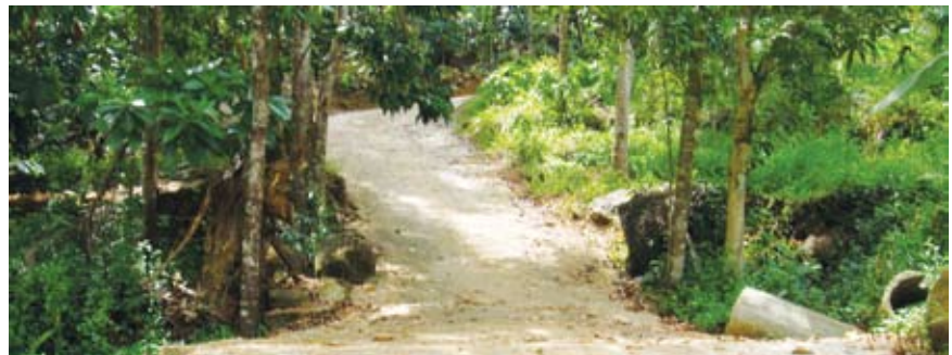
Construction of Access Roads
