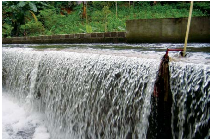
Spillway at forebay tank - Batatota Plant
