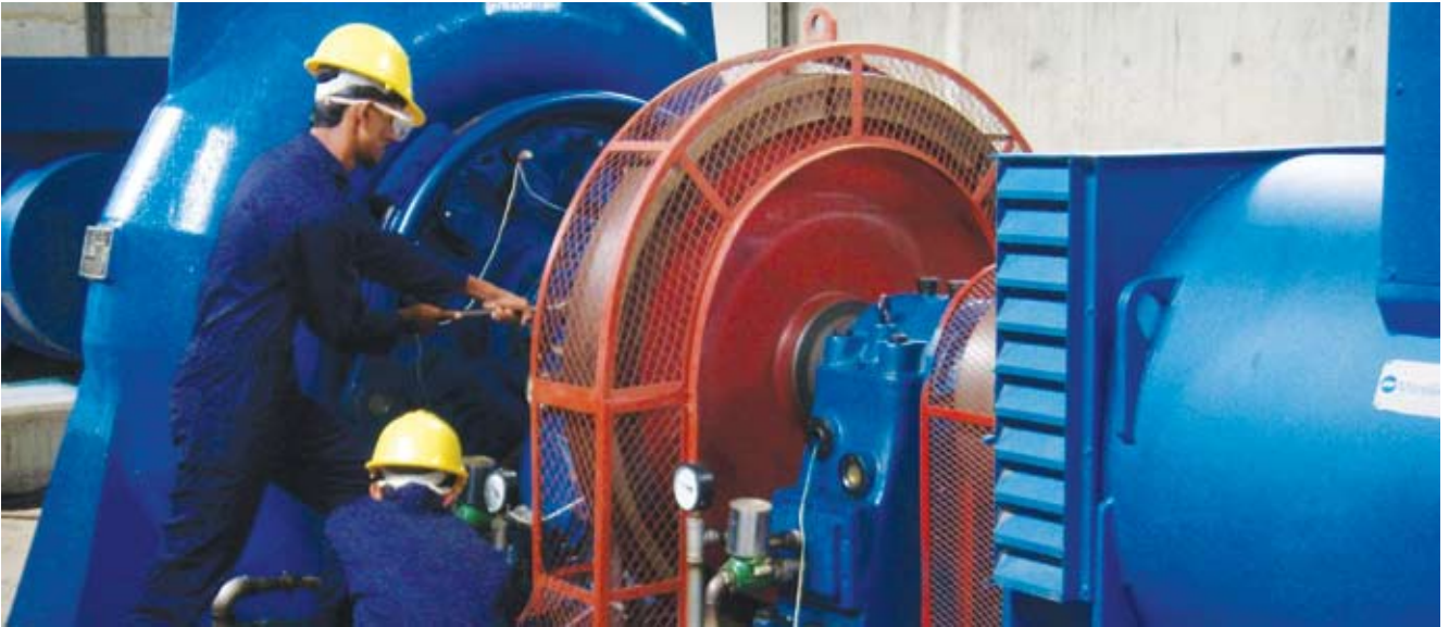
Maintenance of Turbines - Power House - Batatota Plant
