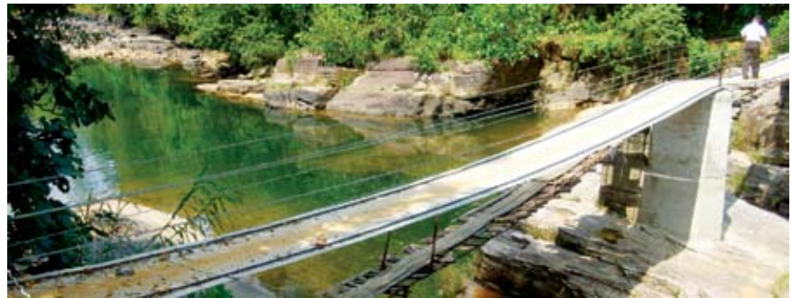
Refurbishment of a suspension bridge
