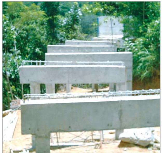
Elevation of the Aqua Ducts - Batatota Plant
