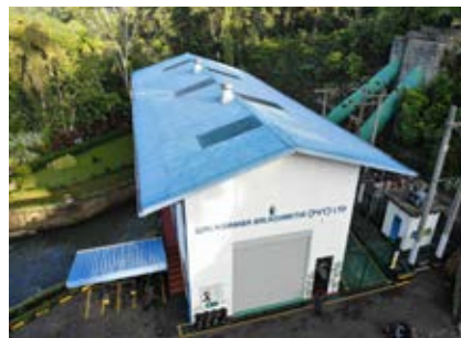
Wembiyagoda MHPP - Powerhouse
