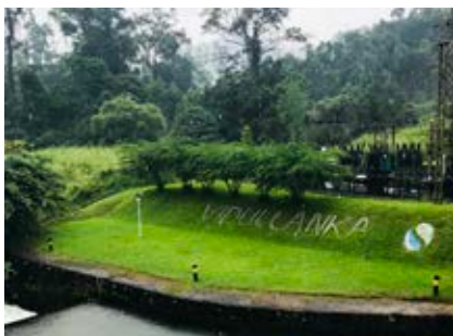
Bambarabatuoya MHPP - Tailrace & Switchyard
