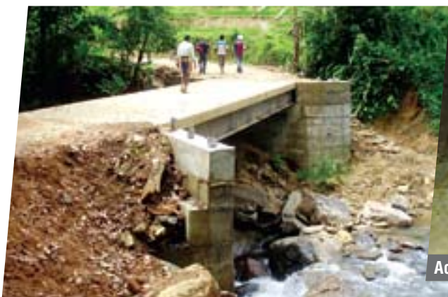
Bridge at Udugama Village
