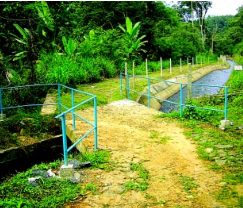
A view of the Headrace Channel A safety crossing for Public
